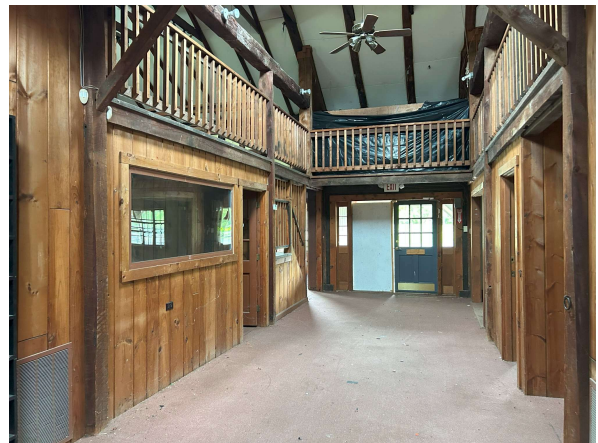
Photo #16 Interior view of the site building
