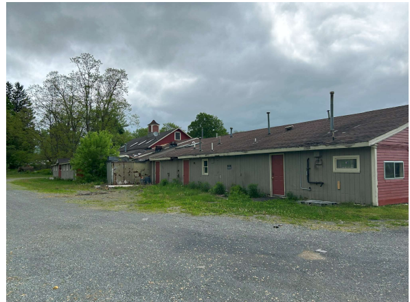
Photo #2 Rear (north) façade of the site building
