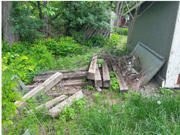
Photo #7 Debris located adjacent to the shed
