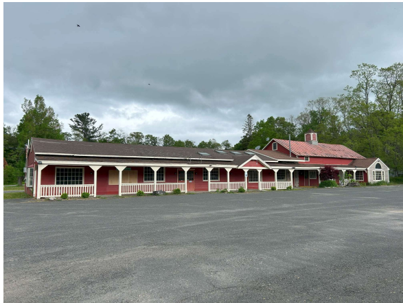
Photo #1 Front (south) façade of the site building
