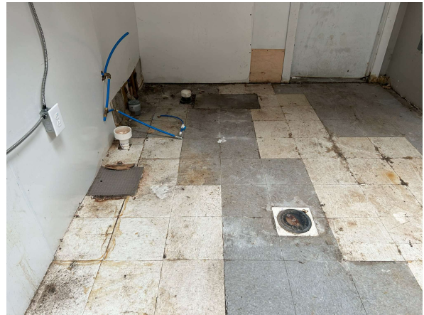
Photo #14 Floor drain located within a former restaurant kitchen area
