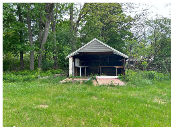
Photo #6 Shed located on the east side of the site
