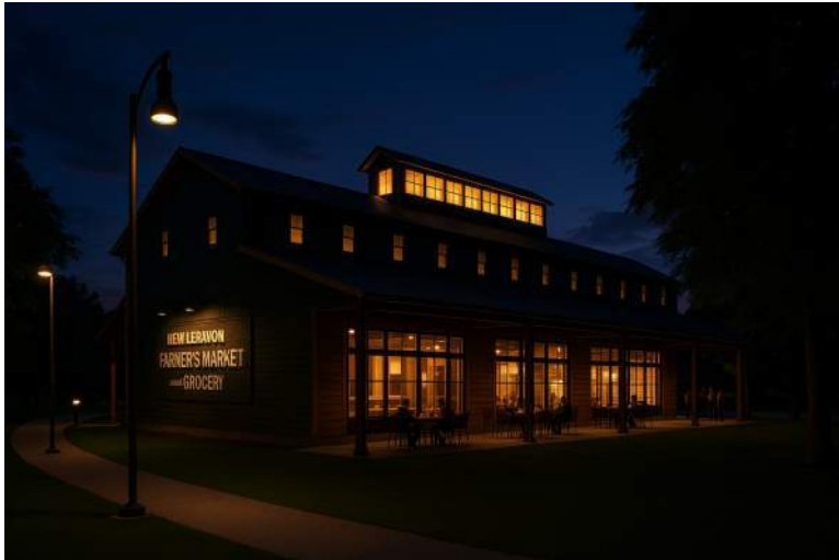
Selux Avanza on 12' pole for pedestrian path, spaced roughly 20' O.C.
